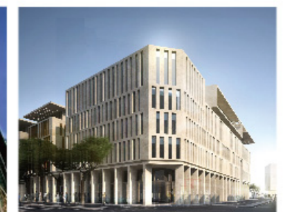
HMODA elevator in Israel
